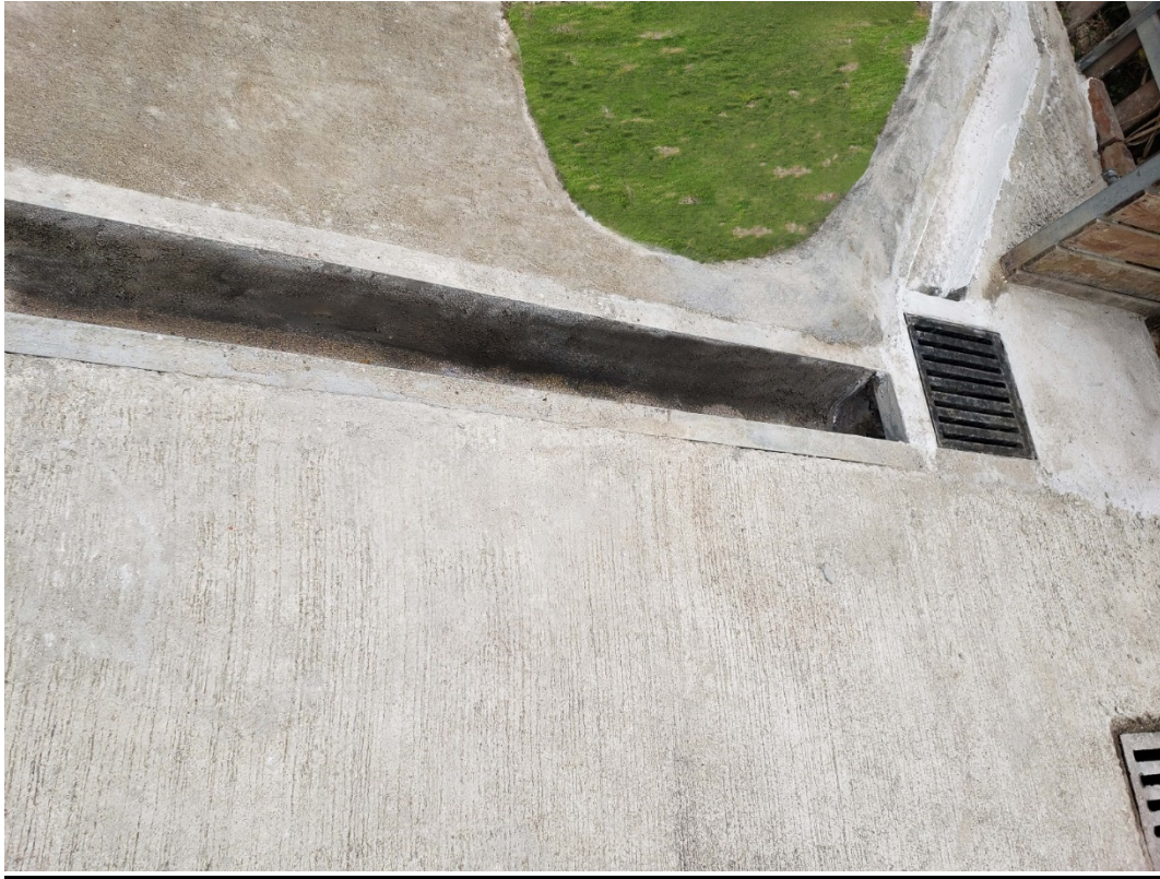
Photo (1) : The terminal catchpit
